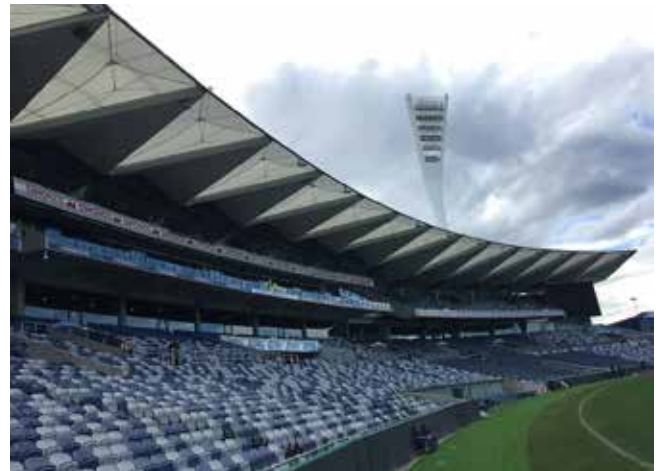
Simonds Stadium Stage 4 – grandstand from inside the arena
