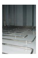
The PPG PHENGUARD 965 three-coat system is easy to apply using standard shipyard methods. It has the same broad range of chemical resistance and outstanding performance features as the market-leading PPG PHENGUARD 930/935/940 system, combined with improved application, curing and smoothness.
