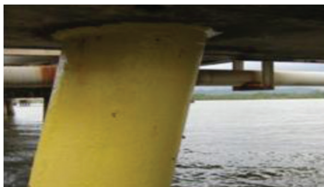
First image: Initial condition
