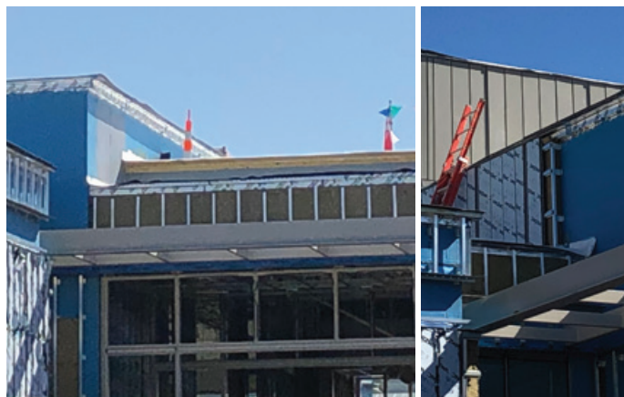
PPG PSX 805 coated exterior steel structures and trusses.
