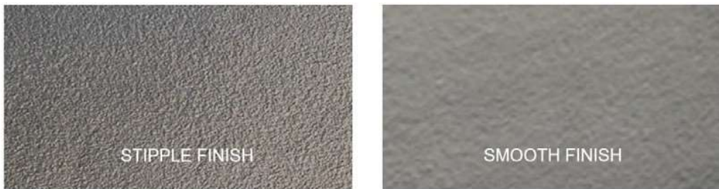
Figure 6: Example of high-quality finish appearance
