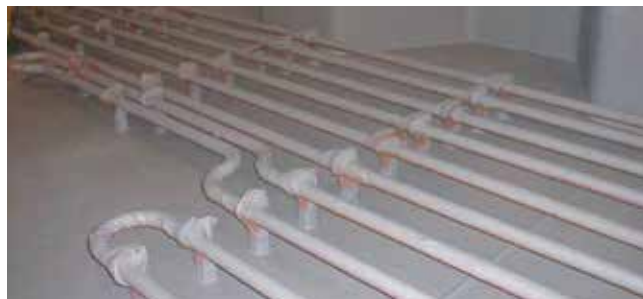
Tank bottom of the Rhonestern after applying 3 layers of PPG PHENGUARD
