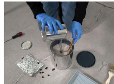
Pour ALL the contents of Part A into the larger Part B container. Mix for at least three minutes. Be sure to scrape the sides and bottom of the containers so that all material is properly mixed.
