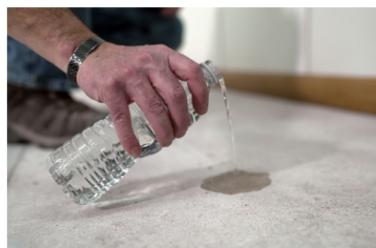
**Remove foreign substances:** Scrape off any putty, paint or oily dirt. Flush the entire area with water.
